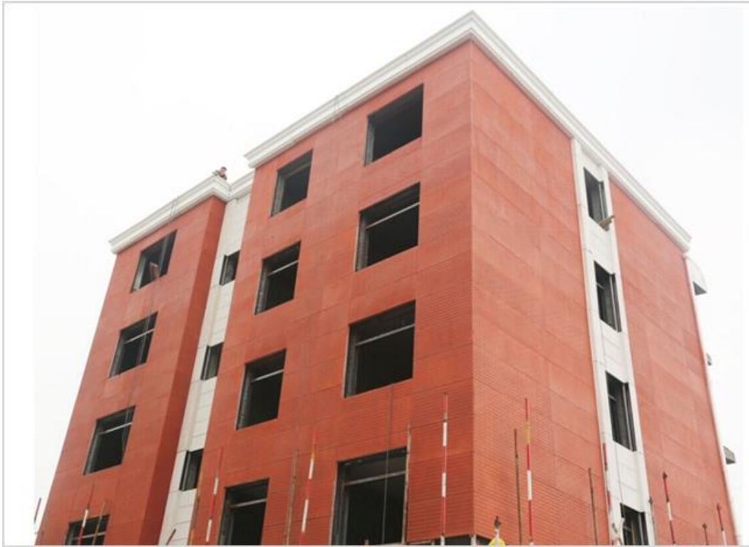
Figure 5: 3D printed building in China (Source: Winsun 7 )
