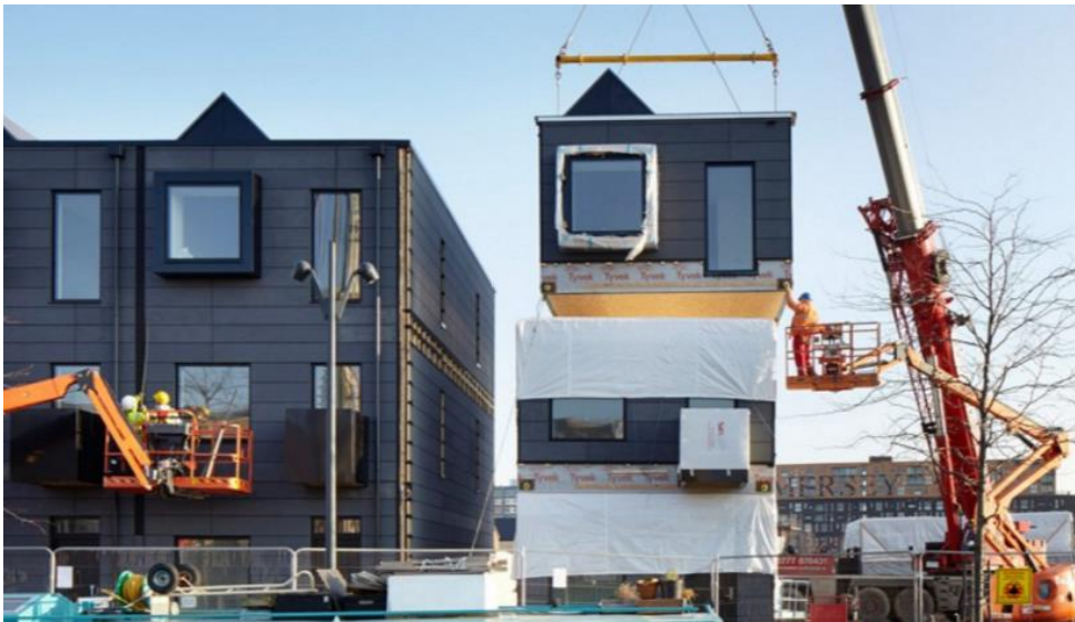
Figure 6: Modular building construction in Manchester (Source: deezen 11 )
