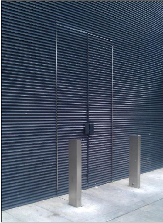
Image showing the external access doors to the waste storage room
