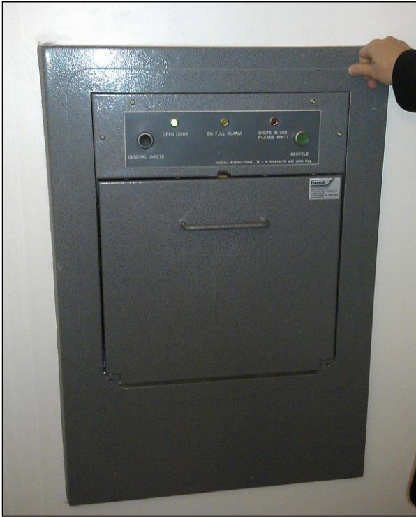
Refuse chute wall panel and access door
